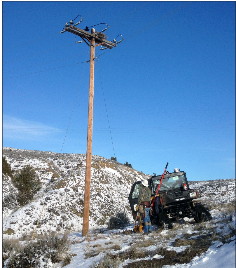
Photo by Manager of Line Operations Gary Kipp. A PRECorp lineman examines a damaged pole.
